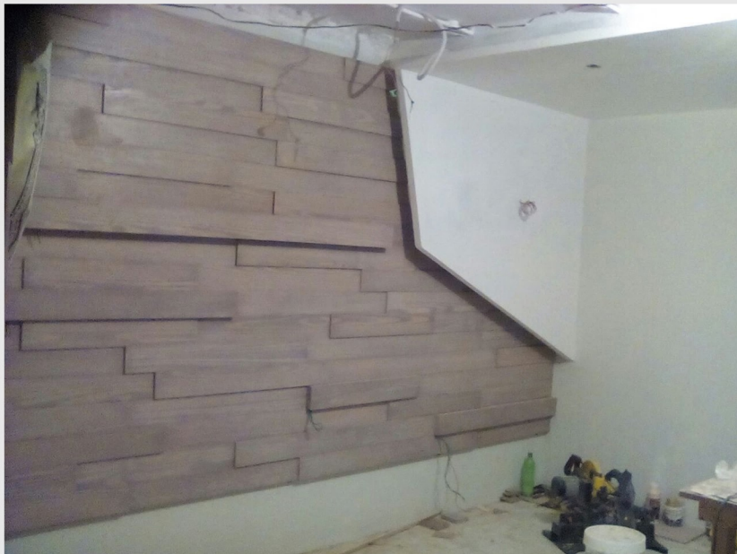
Life shot for the cladding during the installation phase
